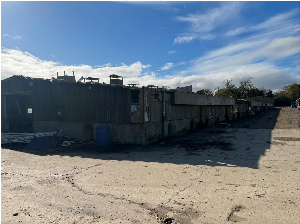
Figure 5: Site of Shed 2
