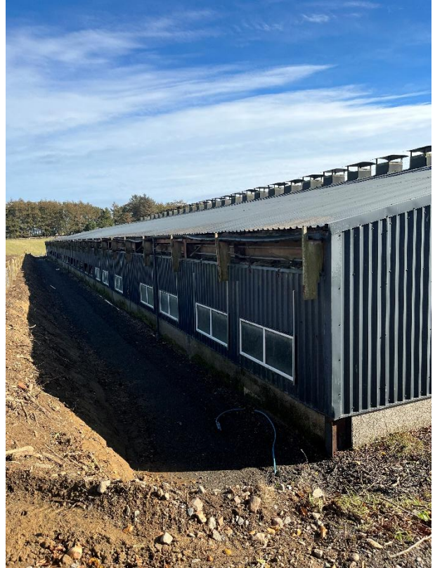
Figure 2: Shed 1 from site entrance
