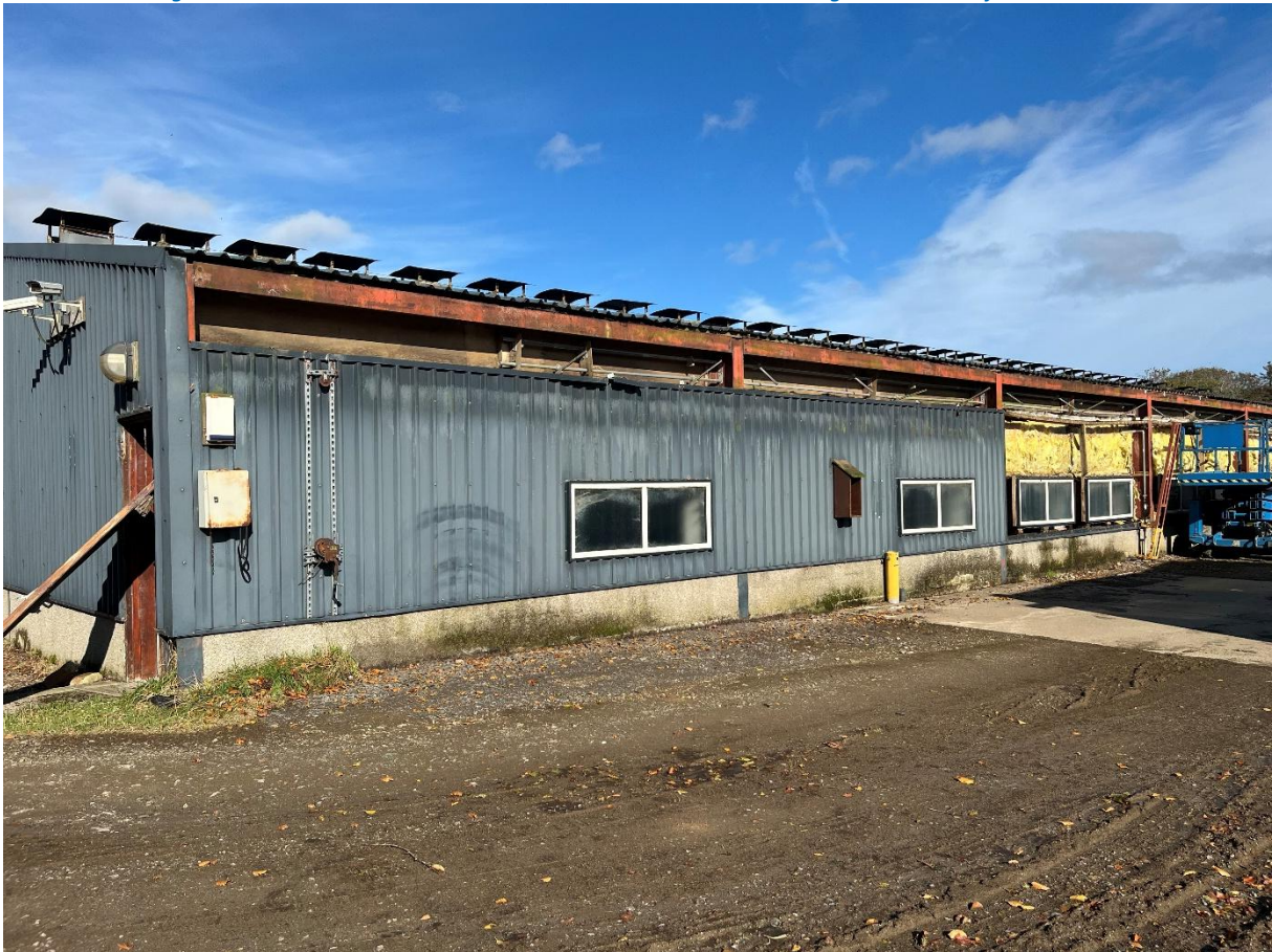
Figure 3: Shed 1 from site entrance
