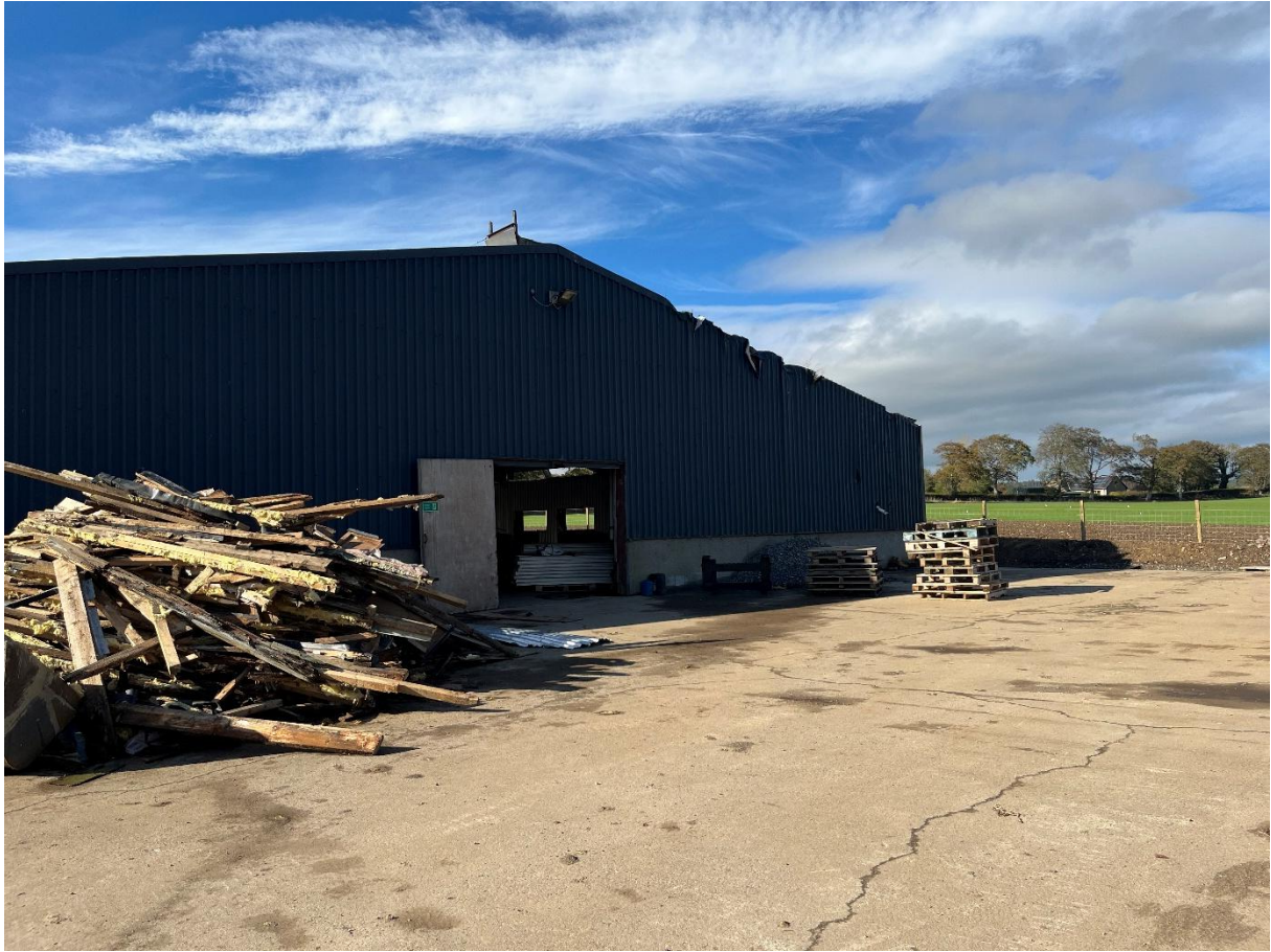
Figure 4: Back of Shed 1
