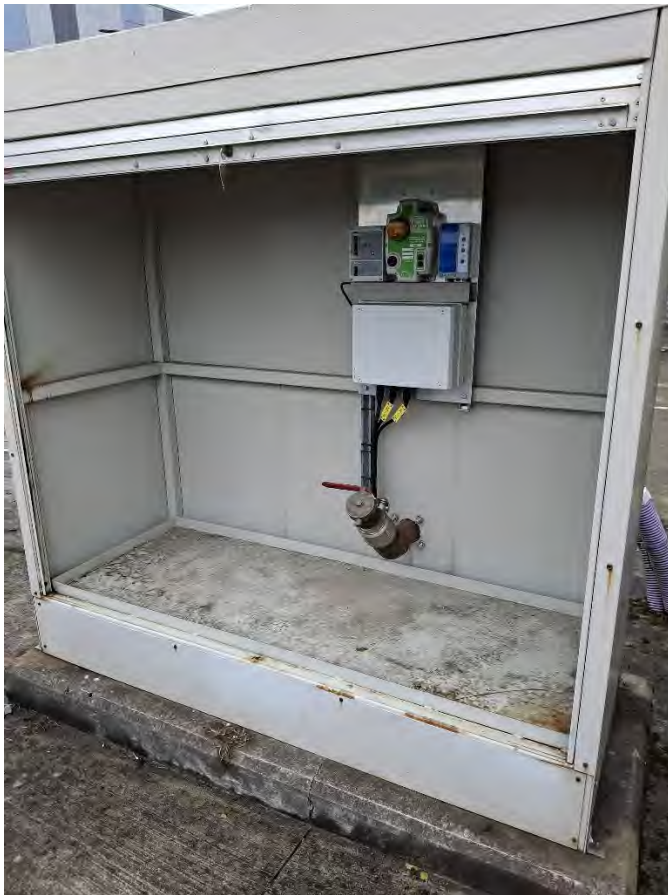
Photo 18 – Meter inside fill point showing how much fuel is stored in the underground tank
