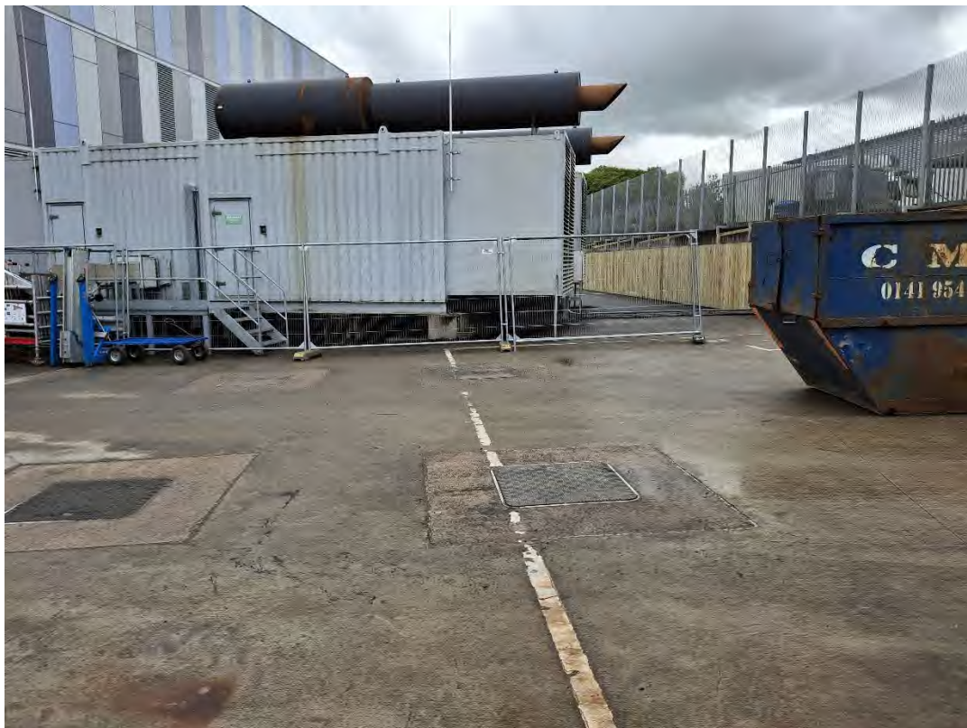
Photo 2 – Looking east toward existing generator and inspection chambers of underground fuel storage tank located inside security fence
