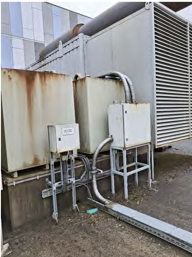
Photo 6 - Looking north, Generator service tanks located between the two existing generators
