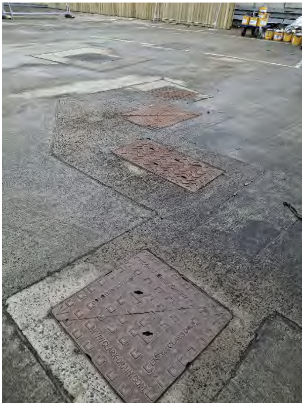
Photo14 - Interceptor inspection covers
