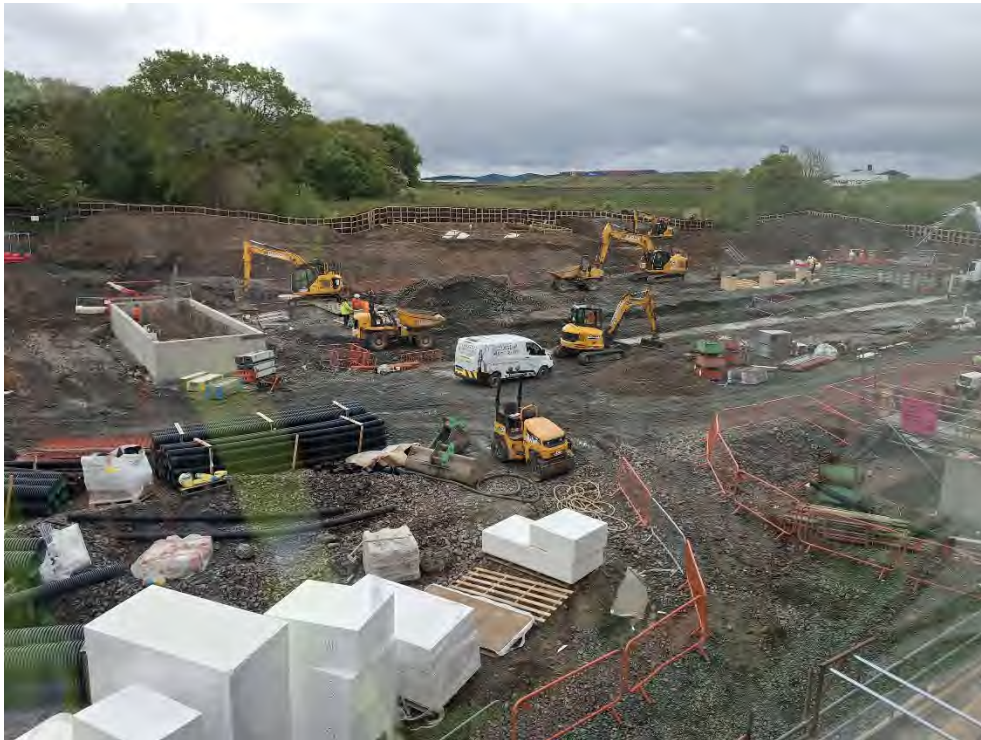
Photo 11- Looking east onto construction site of new generators
