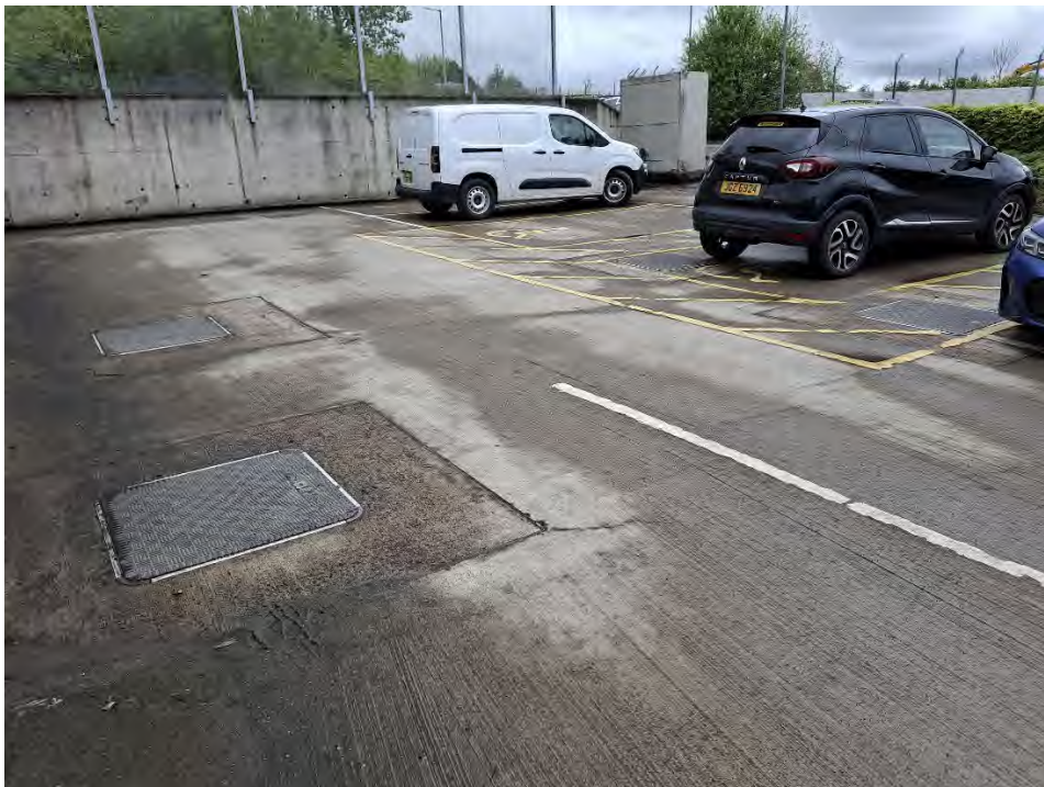
Photo 16 – Inspection chambers of underground tanks located outside security fence
