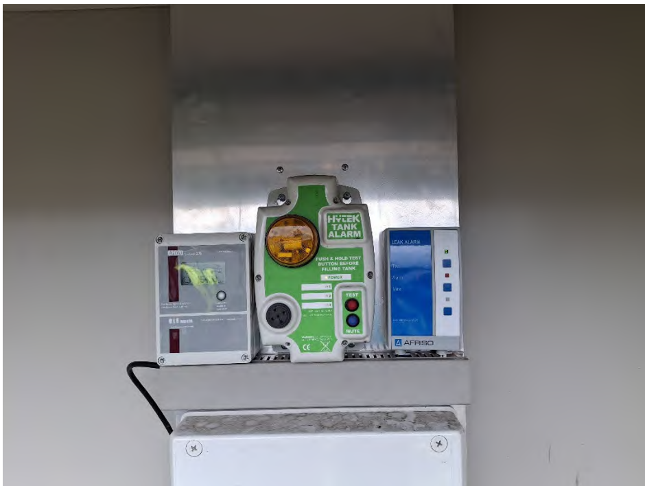
Photo 18 – Meter inside fill point showing how much fuel is stored in the underground tank
