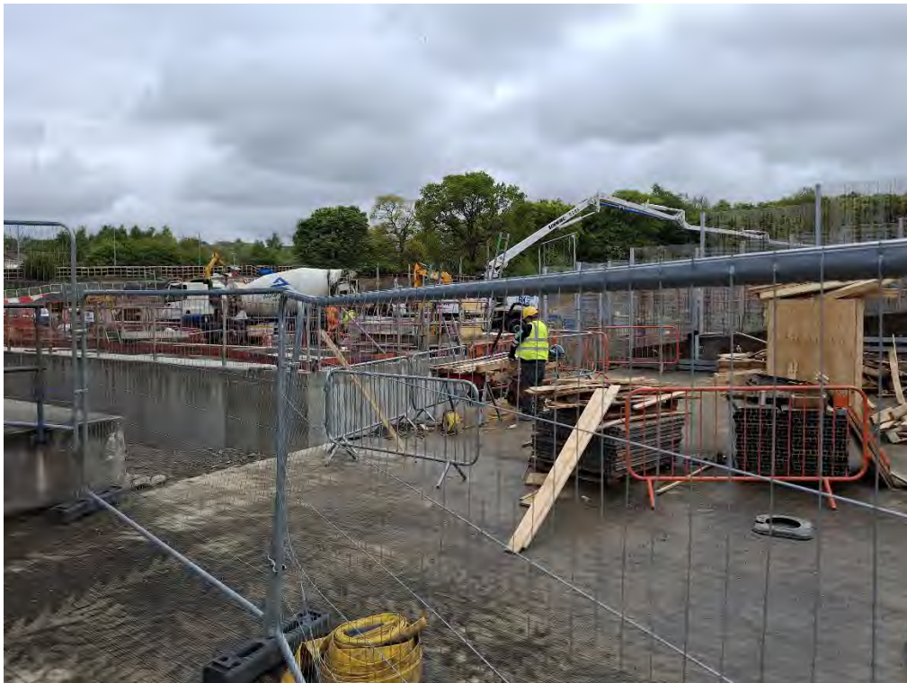
Photo 10 – Looking east toward construction site of new generators
