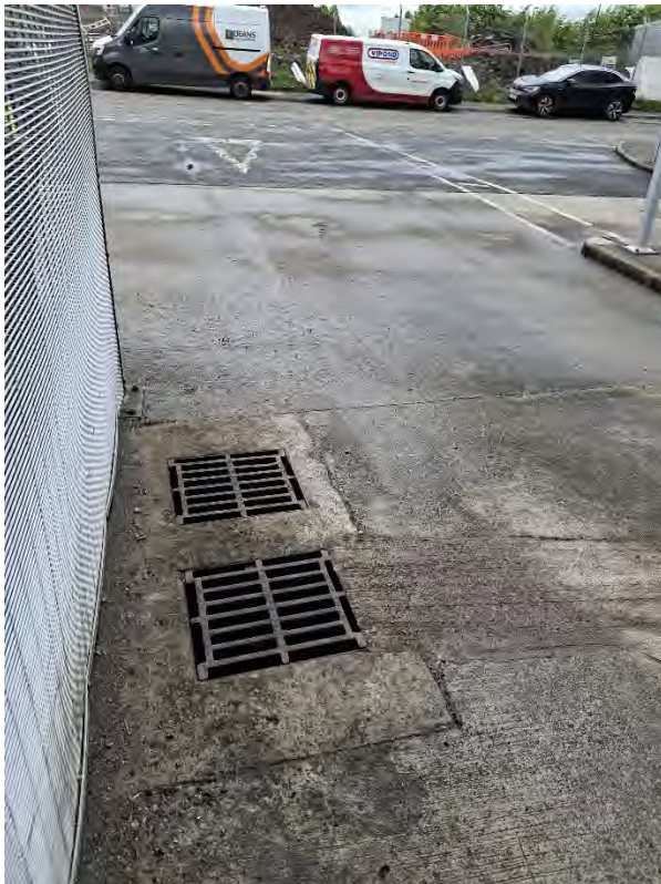
Photo 15 – Surface water drains located outside security fence
