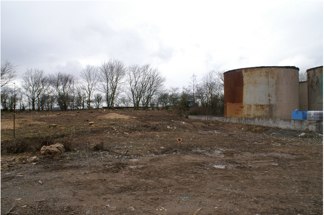
Photo 6 - Looking SW into new land area across unused hardstanding area in existing site.
