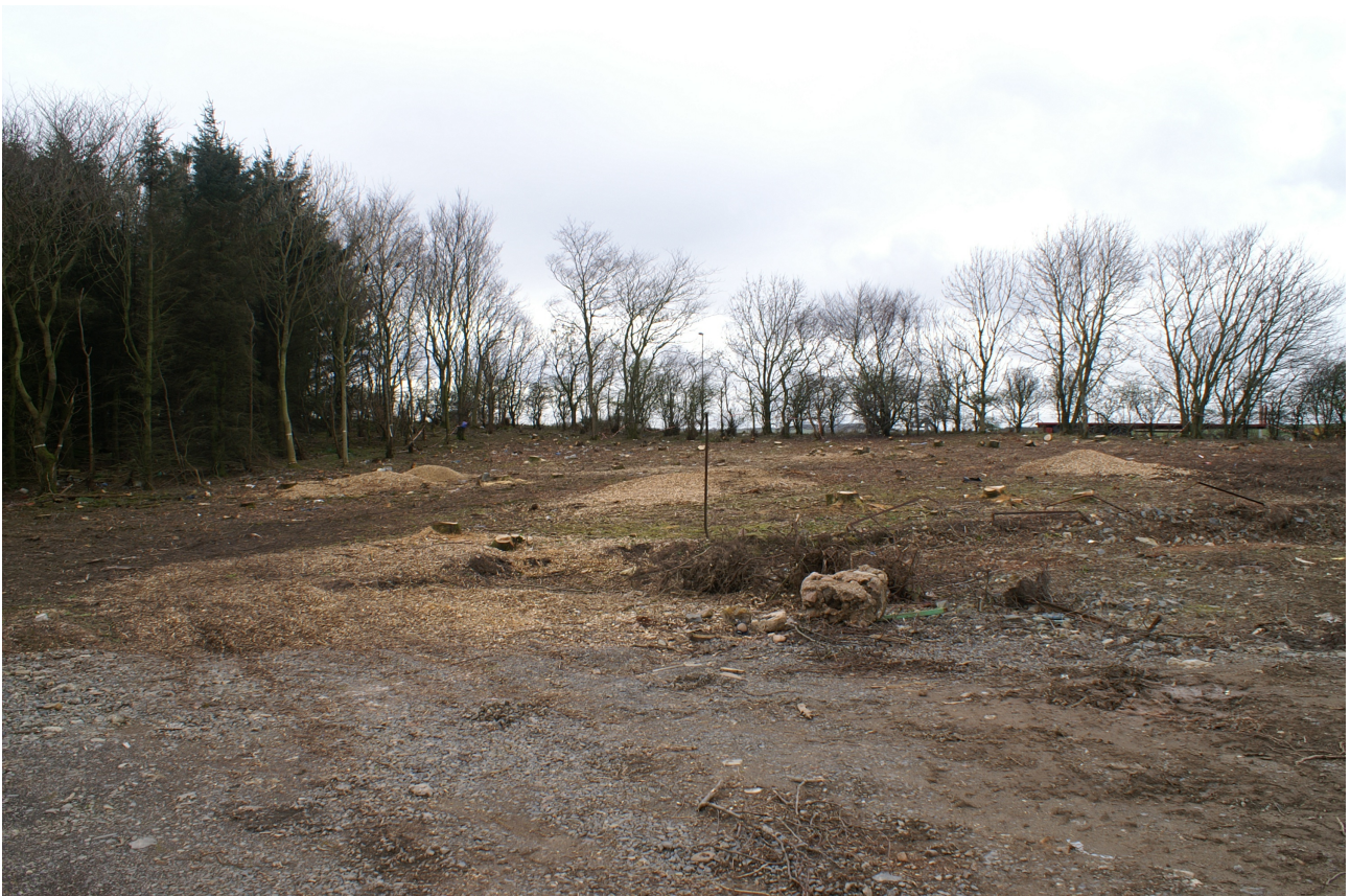
Photo 7 – View of new land area following tree clearance, prior to earthworks to bring down to level of hardstanding area in foreground (boundary of existing site).
