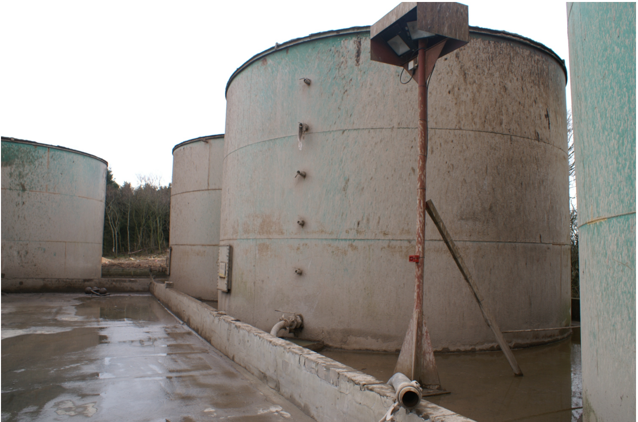
Photo 2 – Existing cuttings / slops storage tanks with bunding. Tanks are open topped and not pressurised.
