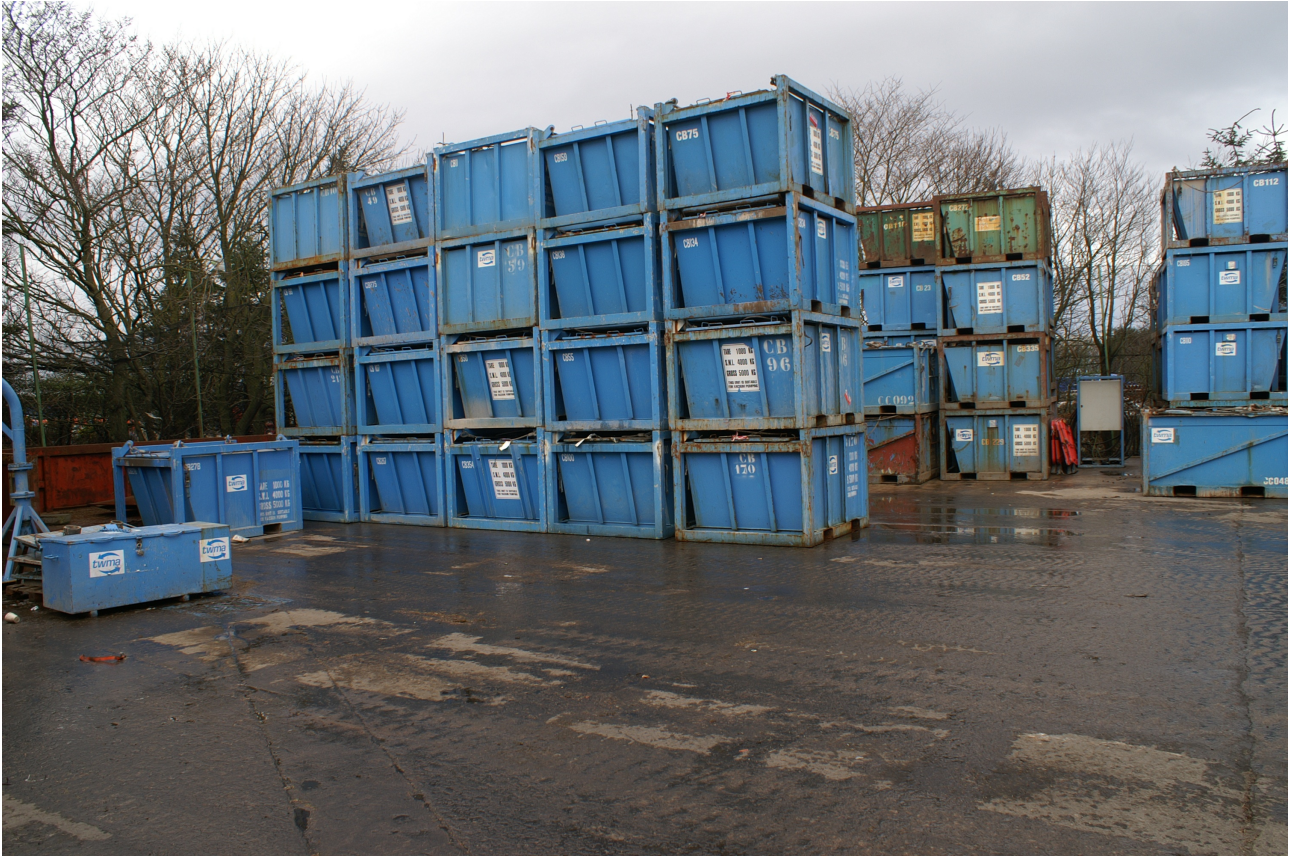
Photo 1 – Existing bin storage area in corner of site, with concrete surfacing. Surfacing has no raised kerbs at edges, but falls into site.
