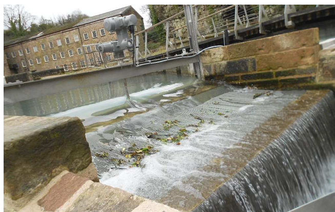
Figure 4 : Tyrolean overwash screen
