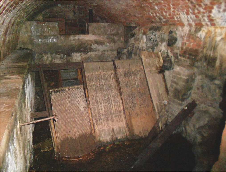
Figure 14 : Forebay tank and fine screens
