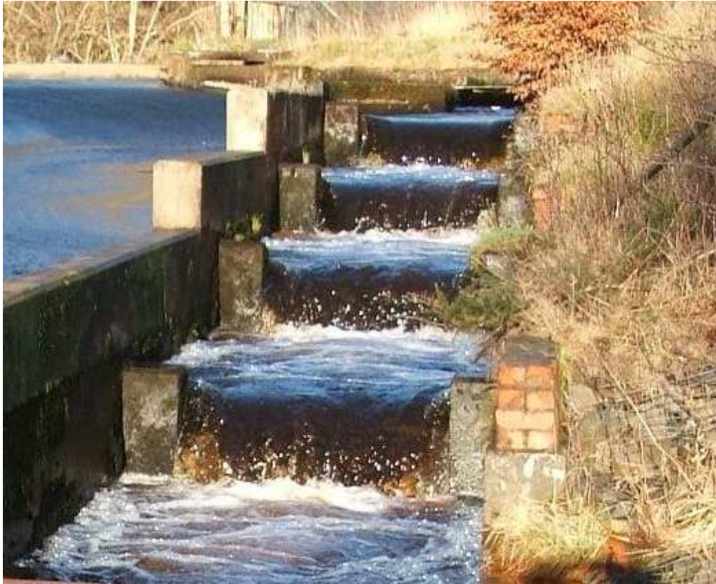
Figure 3 : 200mm passing over the crests of the fishpass
