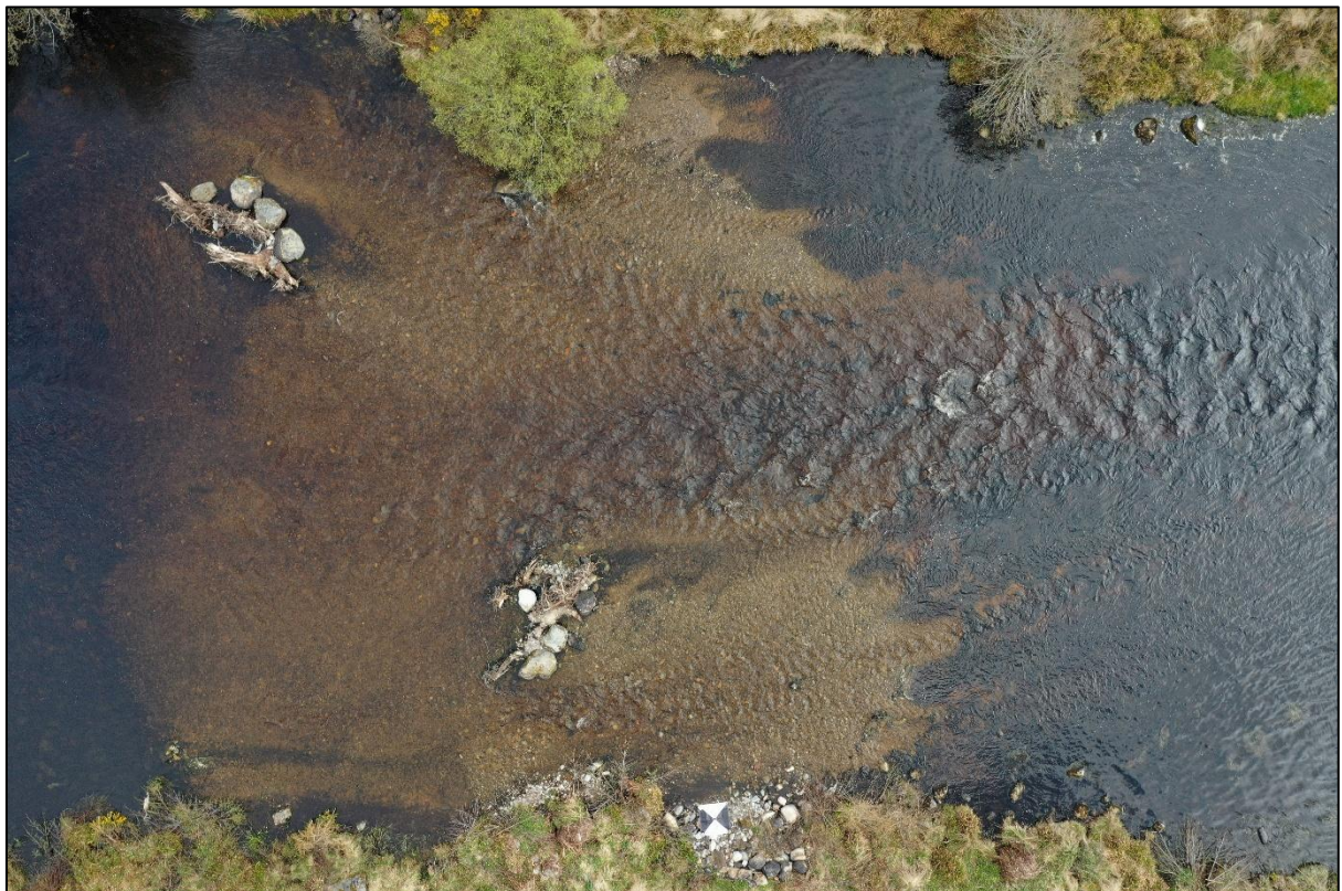
Figure 1. Example of gravel augmentation/ LWS works on the River Shin, downstream of the HP dams.
