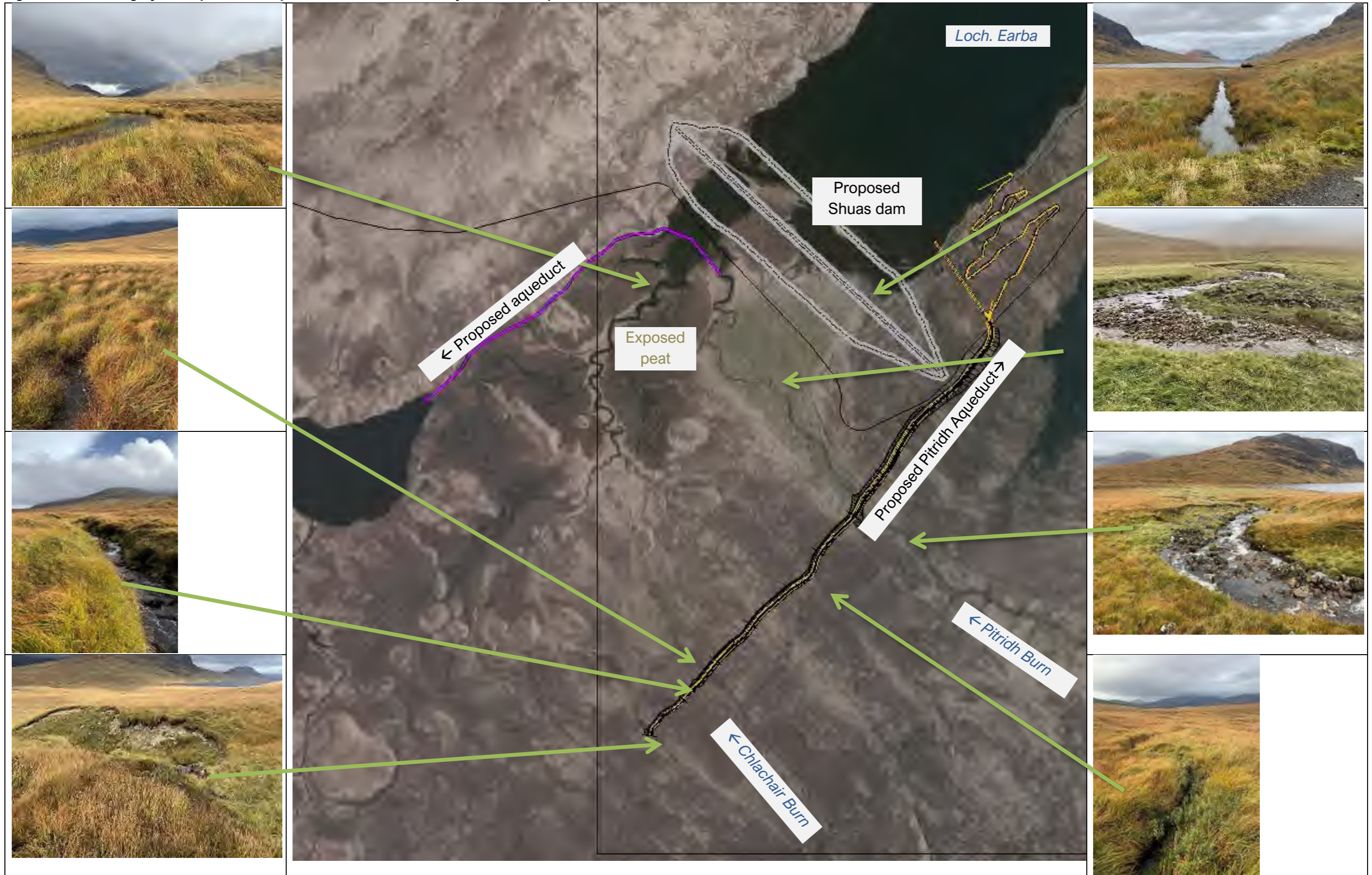
Figure 3-2: UAV imagery and representative photos of the area affected by the Pitridh Aqueduct
