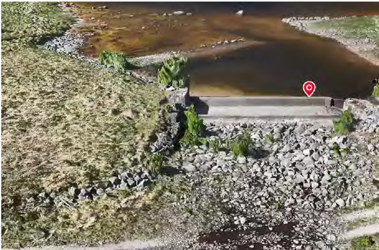
Figure 5-1: Sediment distribution upstream of the existing Loch Earba outlet
