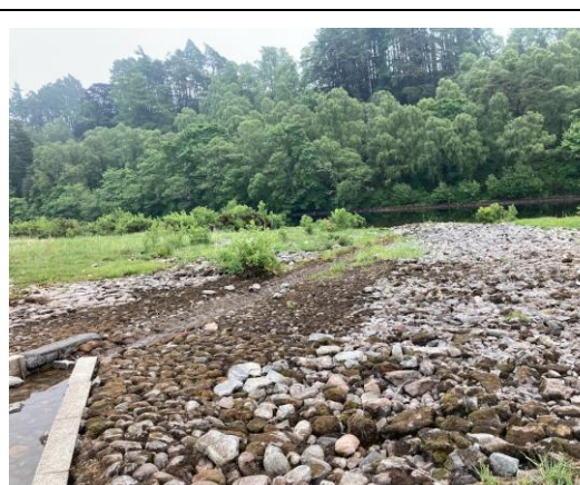
Plate 13.2: Smolt chute flowing towards the River Ness with minimal flow and water depth across the waste weir during low loch levels.
