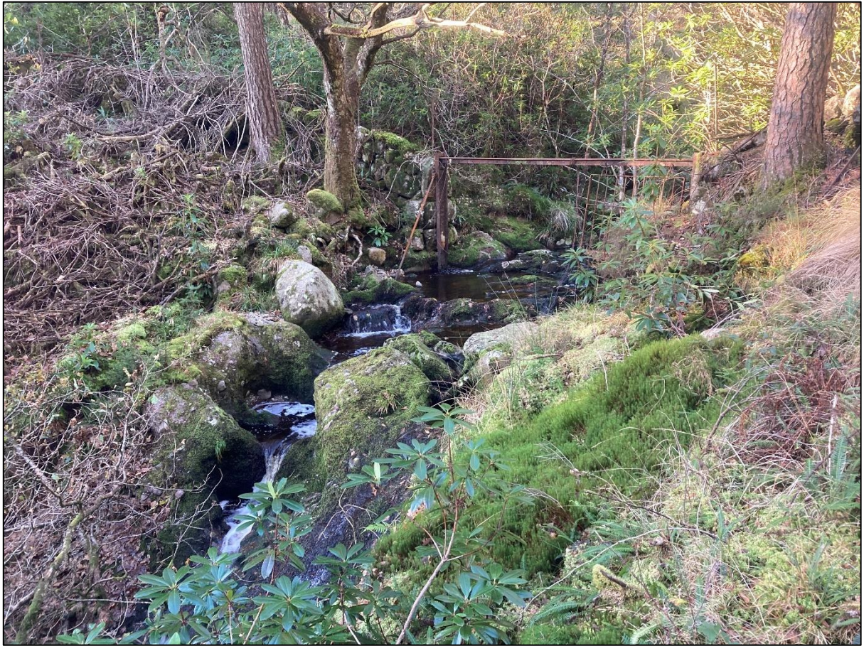
Figure 3.14. Old gate over channel
