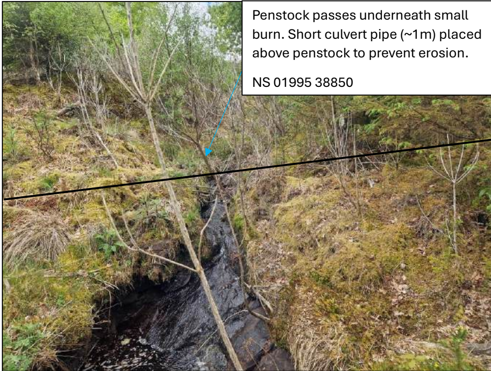
Figure 23 – New culvert at NS 01995 38850. Penstock still within ATV track
