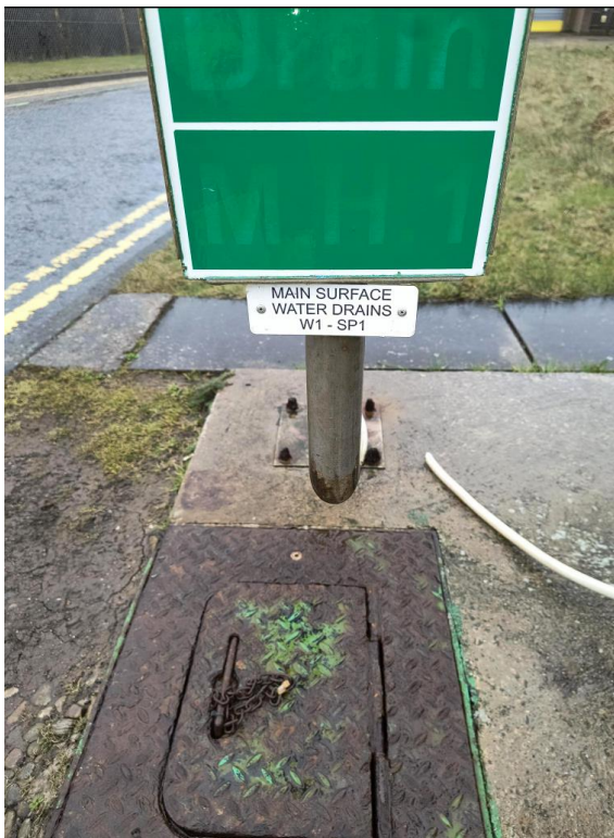
Photograph 1: SP1 Located at Manhole 1
