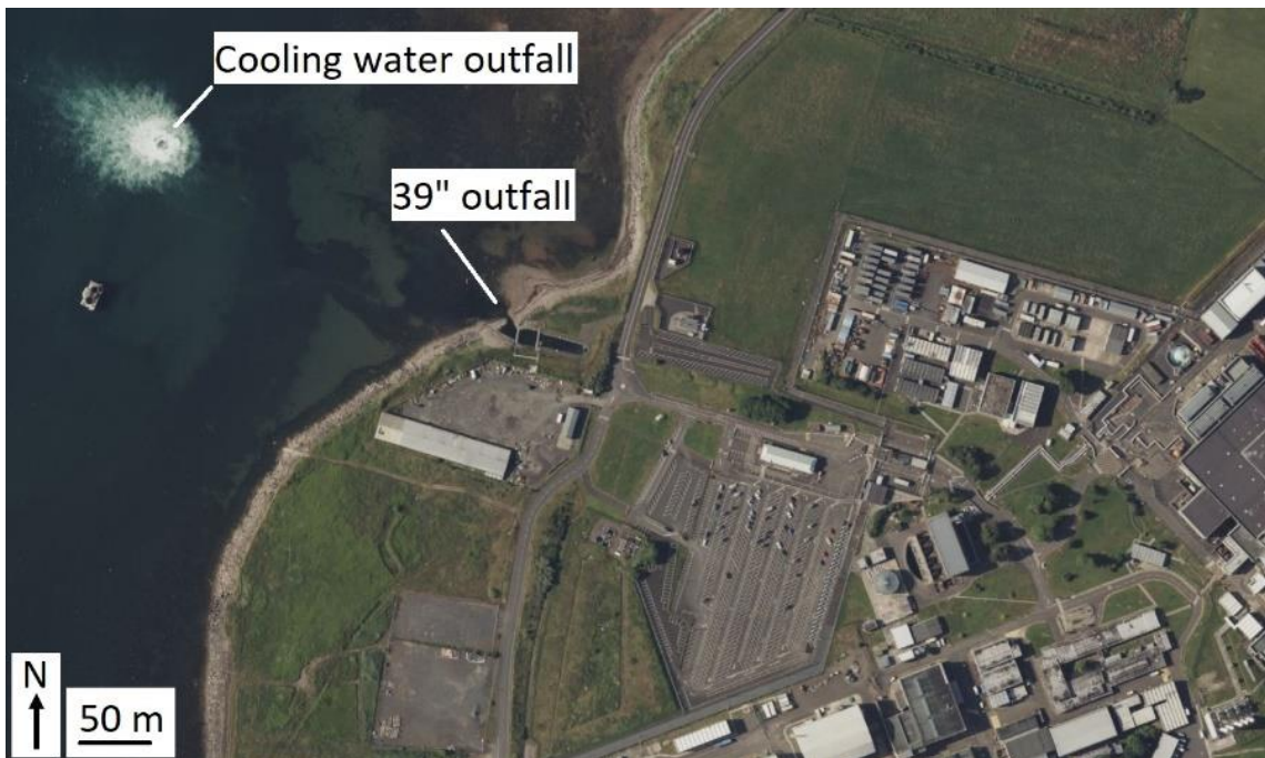
Figure 60 – Aerial photograph showing location of cooling water outfall and 39" outfall (base photograph from reference [39])
